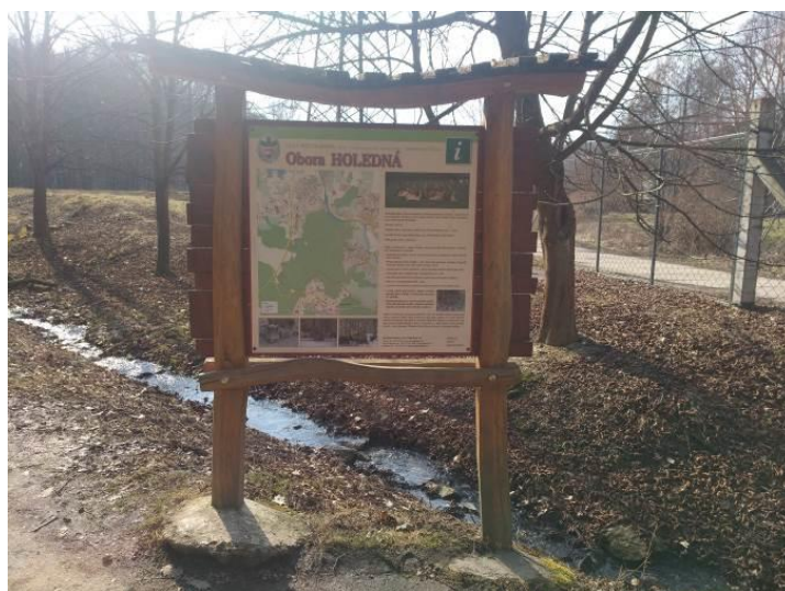
Fig. 2: Unightly concrete footings for anchoring the educational board (Kotásková)
