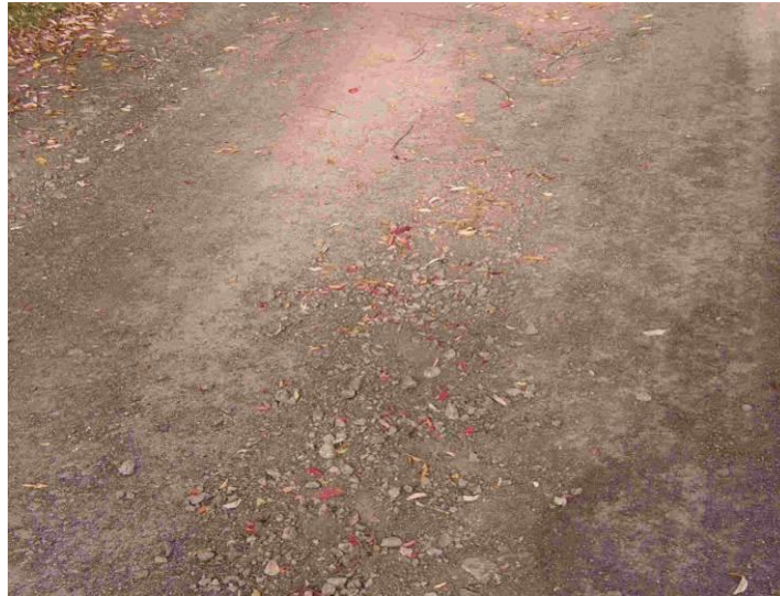
Fig. 1: Detailed view of the modified road cover.
