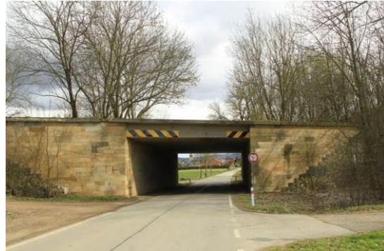
Fig. 3: Bridge over road W of Jevíčko
